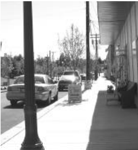
The 7-foot sidewalk along Cherry Street was replaced and widened to 10 feet.
