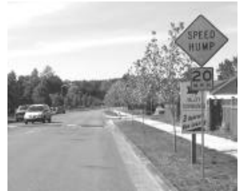
Speed humps were installed on Rivergrove Drive to slow traffic.
