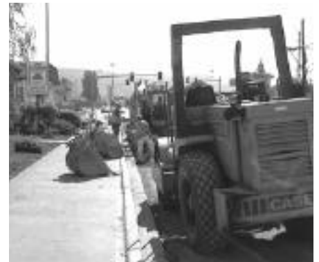
Construction of trunk line on Main Street.
