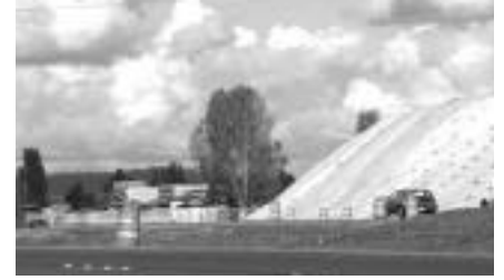
The SR 167 overpass is taking shape.
