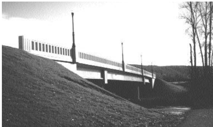
The new bridge over the Stuck River connects 142nd Avenue East with Tacoma Avenue.
